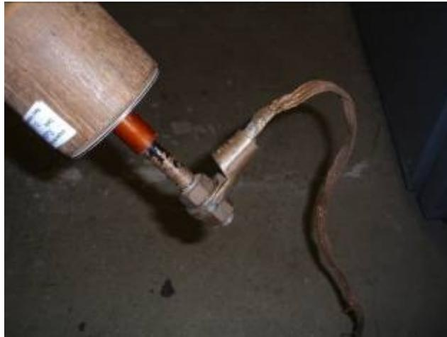
*Figure 5.4C – Earth Connection Applied First to Bottom*
