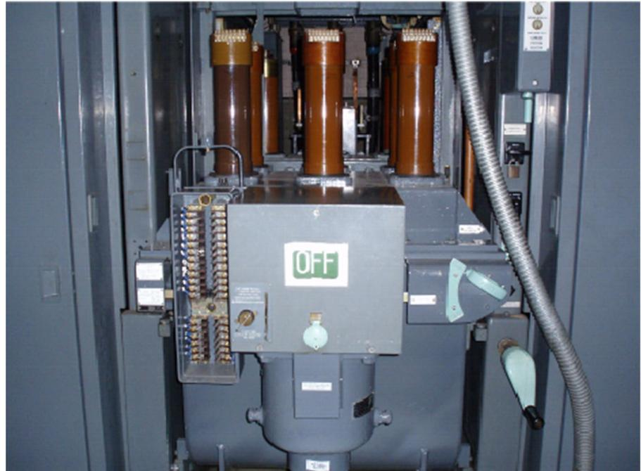
*Figure 7.4A - OCB Withdrawn and Umbilical Removed*
