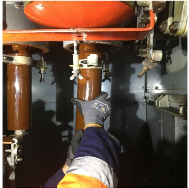
APPLY TEST BUSHING SECURING BOLTS (2 OFF ADJACENT TO EACH OTHER) TO EACH SPOUT FLANGE I.E. 6 OFF SECURING BOLTS.
