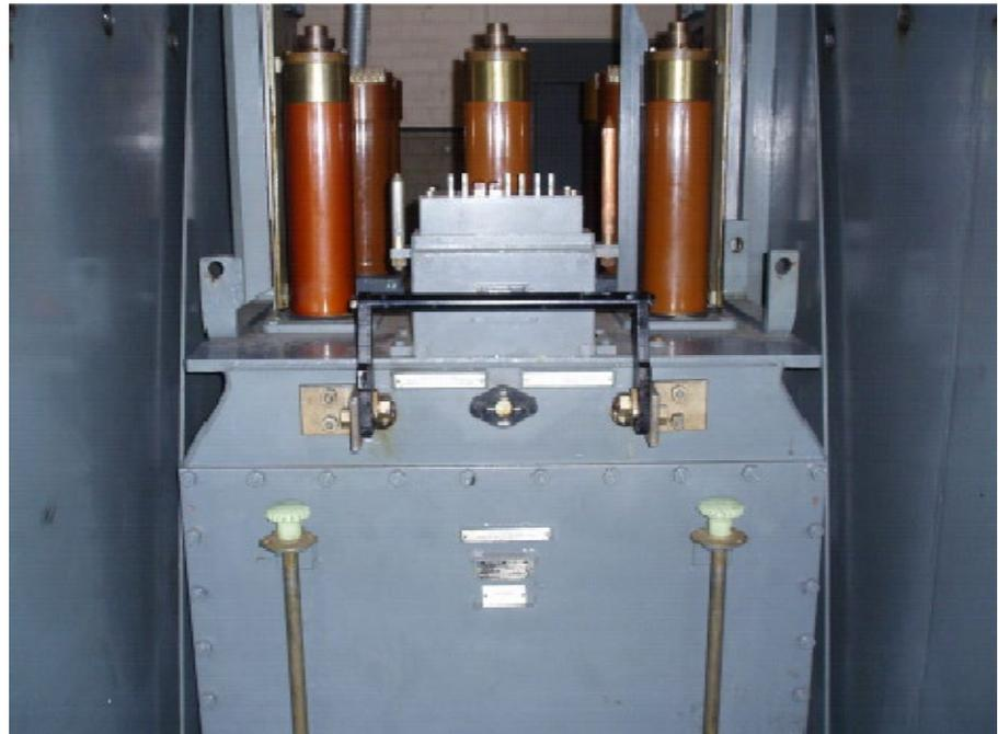
*Figure 7.4B - Voltage Transformer Withdrawn*
