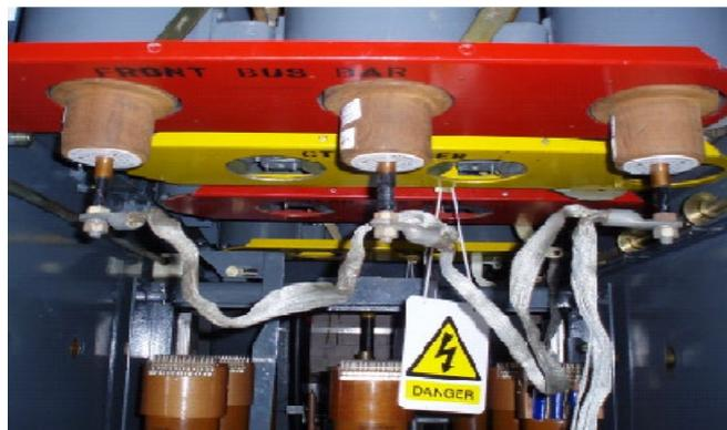
Figure 5.4A – **Metal Enclosed Switchgear Moveable Earths**
