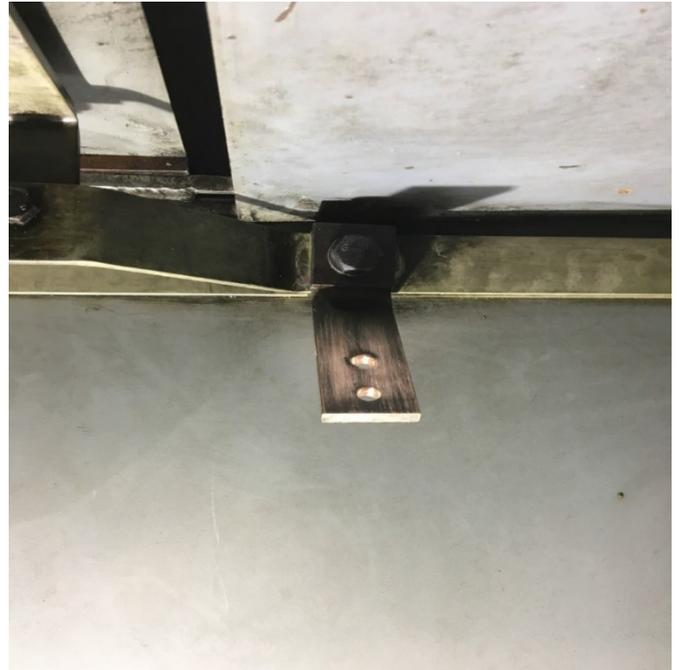
PREPARE 3 OFF 150mm<sup>2</sup> PORTABLE PRIMARY EARTHS WITH EARTH CLAMP AT EACH END. APPLY 3 OFF
