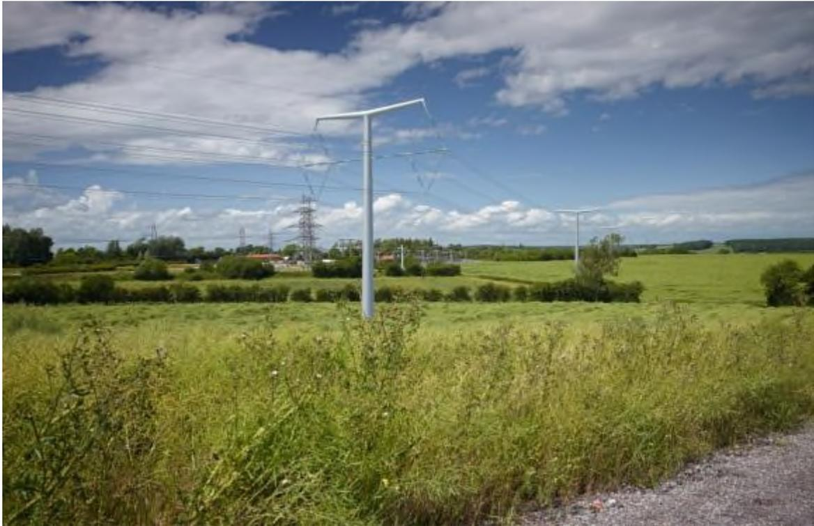
**Figure 5.3 Example low-height pylon**
