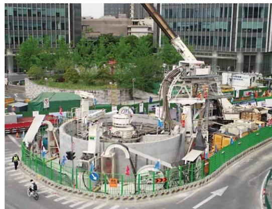
Fig 3 - Herrenknecht VSM showing compact site set-up as proposed on Grain-Tilbury.
